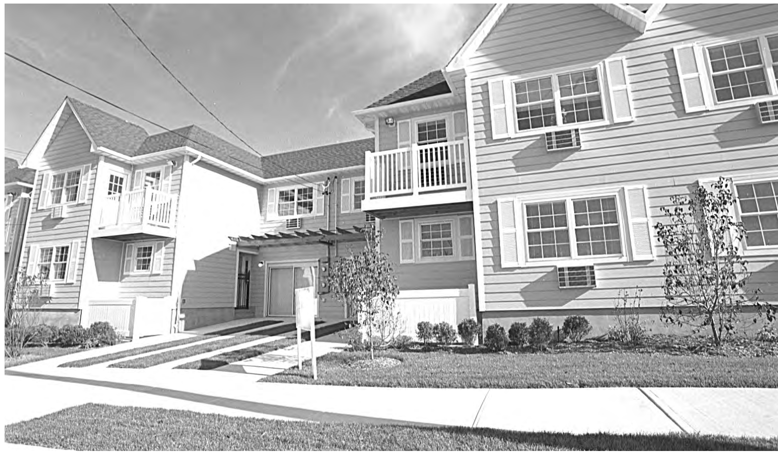
Exterior of finished units
